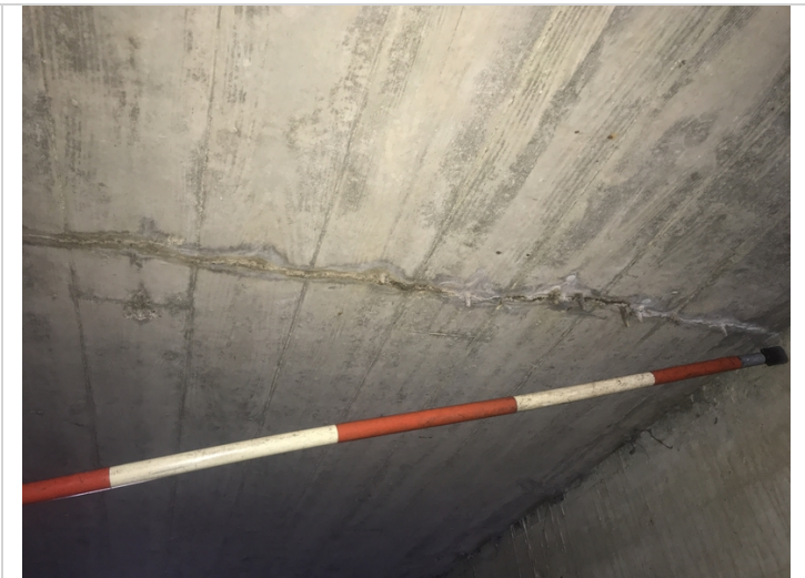
Top of barrel 2 has cracks with efflorescence.
