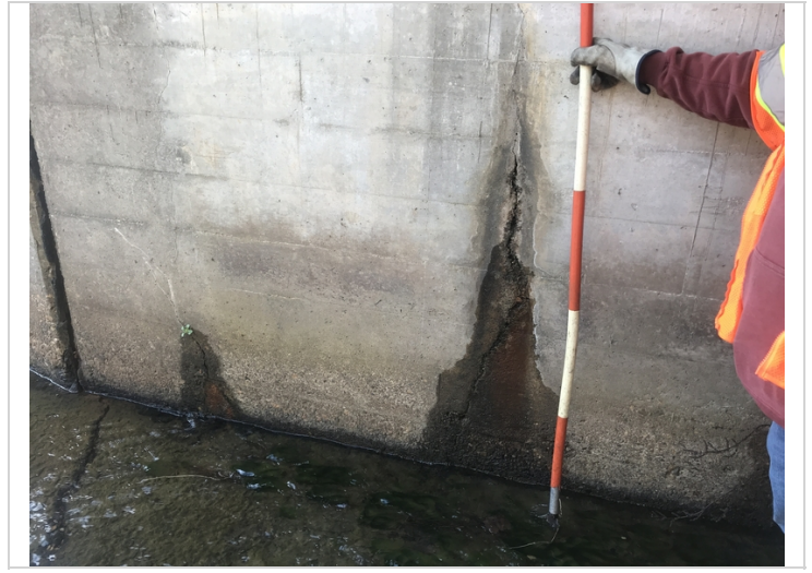
Barrel 2 outlet end has crack in wall. Common along both barrels.
