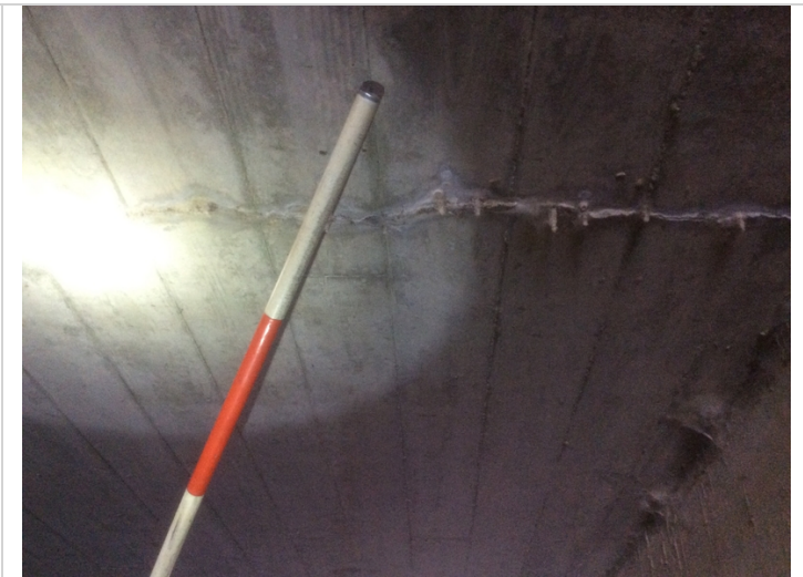
Cracks with efflorescence in the top of barrel one.
