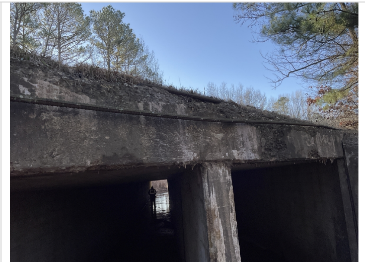
Inlet end with spall and exposed rebar
