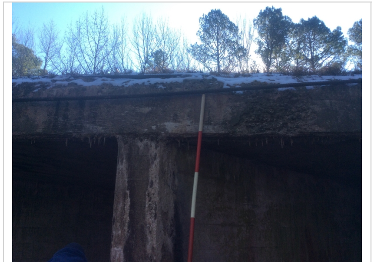
Deterioration to head wall on inlet end of box with exposed rebar.
